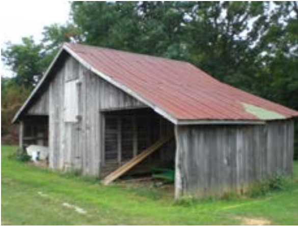
Figure 2.13: North facade of shed (Structure #5)
