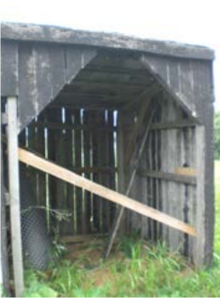
Figure 2.9: Pump house (Structure #3)
