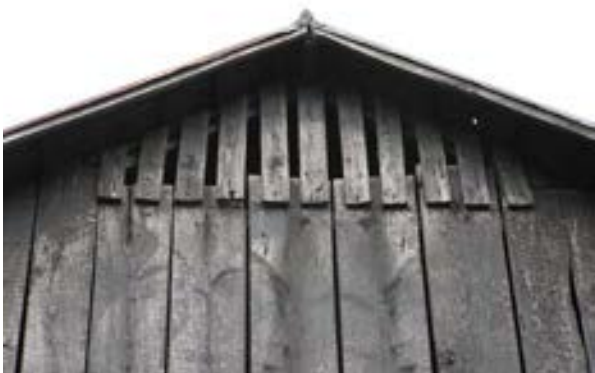
Figure 2.7: Detail of east facade
