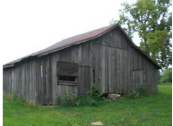
Figure 2.14: South facade of shed; salvaged materials can be used to renovate this small structure in order to preserve an element of the original farm character
