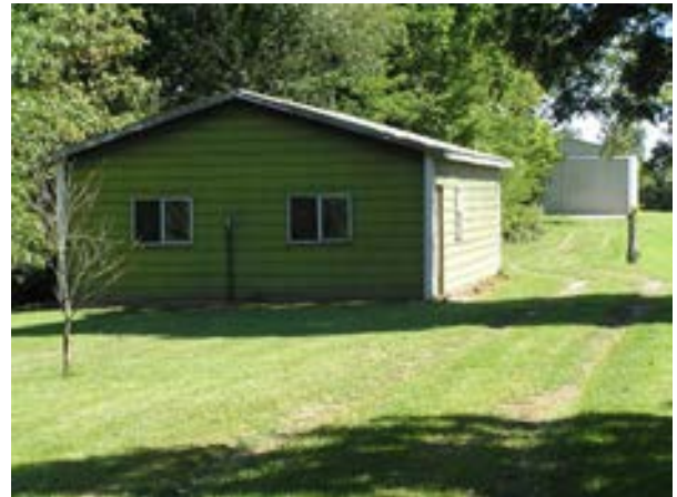
Figure 2.16: South facade of 33'x28', green, metal shed (Structure #7); this building is in good condition and proposed to become the "Bow Hut"--the gathering place and storage area for the archery program
