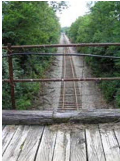
Figure 2.19: Water line tied to bridge railing
