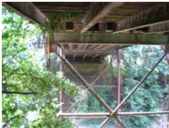
Figure 2.21: Under side of bridge
