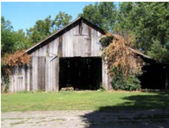
Figure 2.11: East facade of shed (Structure #4)
