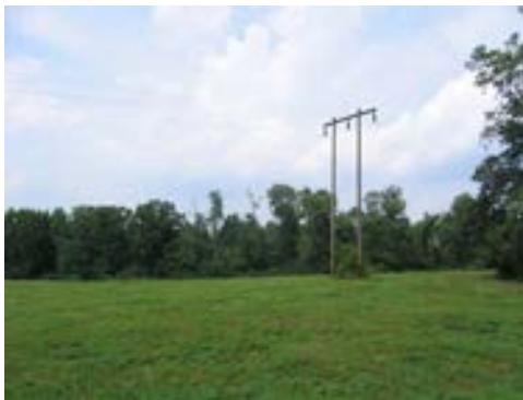
Figure 2.25: Overhead electric line located on the north side of the farm.
