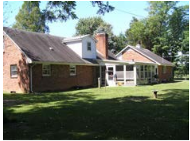
Figure 2.18: North side of the brick house
