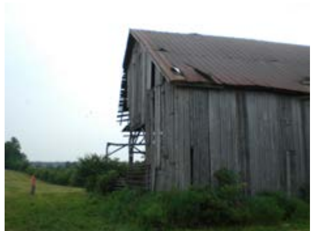
Figure 2.4: Northwest corner of hay barn
