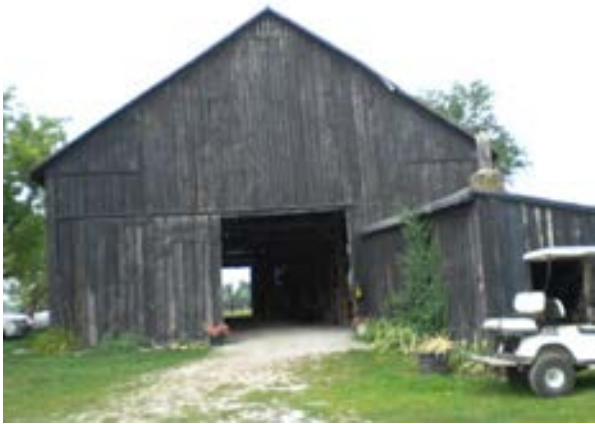
Figure 2.5: East facade of horse barn (Structure #2)
