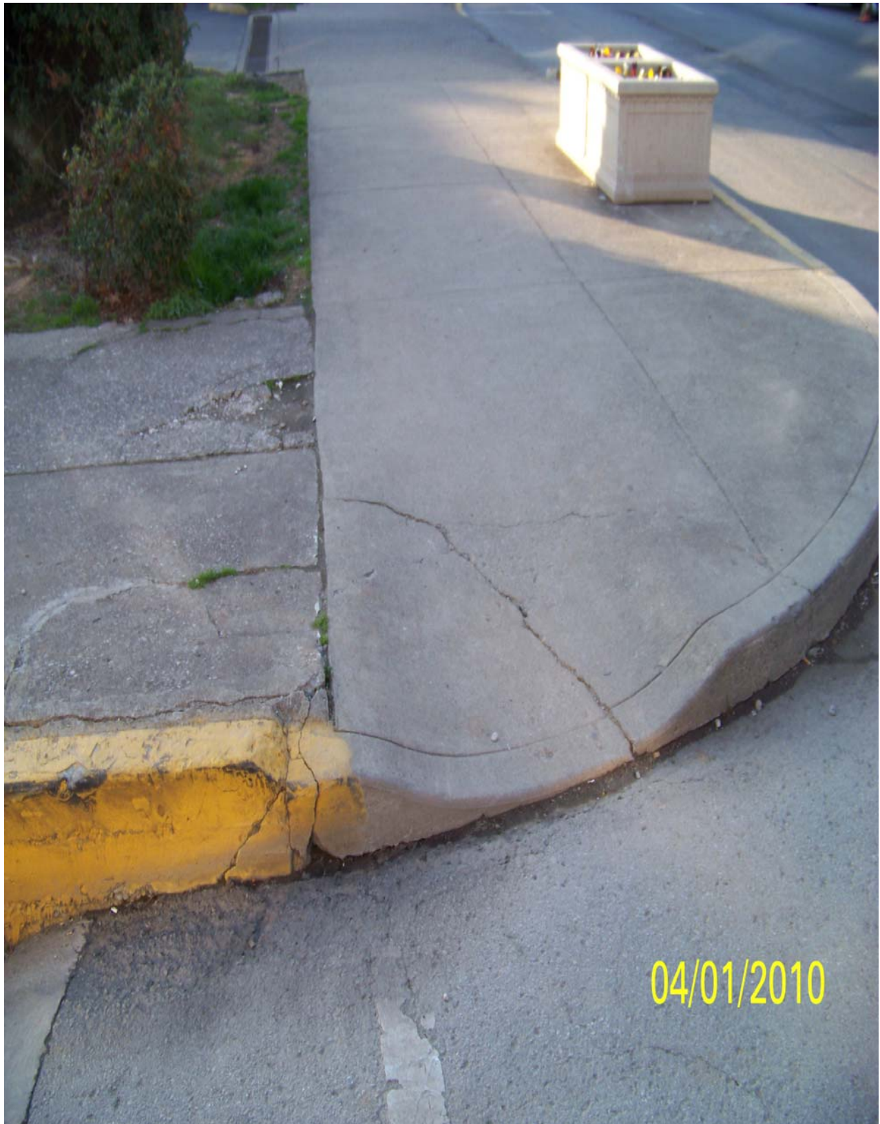
(A) DAMAGED CURB CUT AT MARKET STREET AND SHORT STREET, LEXINGTON
